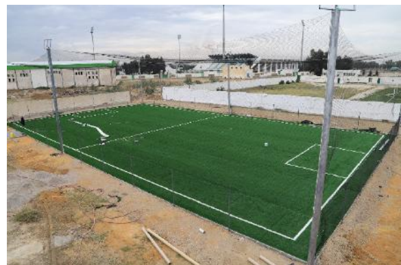
This is the Kairouan Sport Complex after USAID finished its rehab efforts. Photo Credit: USAID.
